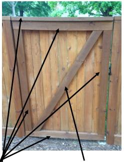
2x4 rectangle framing with inside Z support. Measure from bottom to just below top horizontal 2x4
